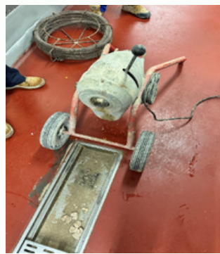
Pic4: The fat went inside the drainage which led to blocked pipes, bad smell, and many hours of maintenance which disturbed the kitchen operation.
